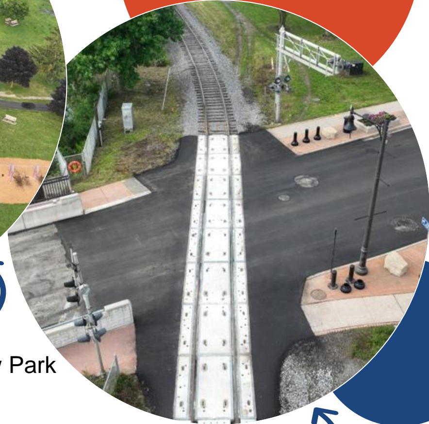
Main St Rehabilitation
