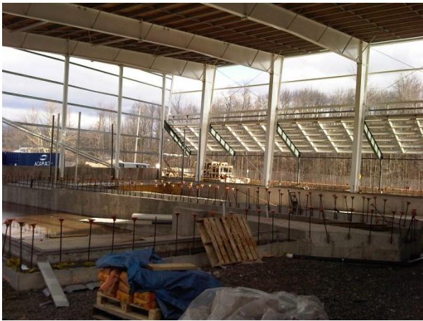
Aquatic centre Steel erected and wood decking is installed
