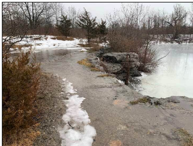
Photo 3. Intermittent Drainage Feature where it outlets (cascades) into the Northern Quarry Pond (17 February 2022).
