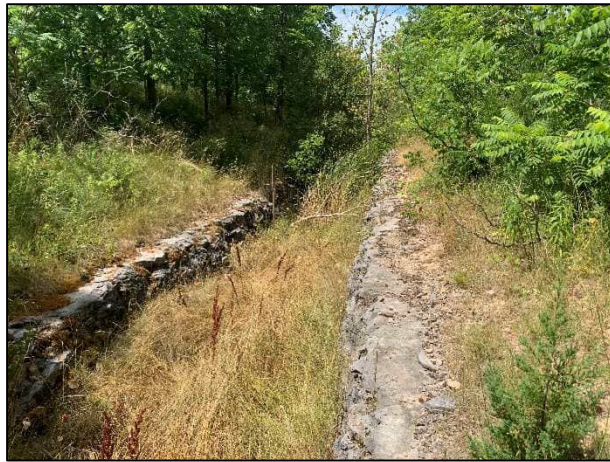
Photo 17. Drainage Ditch within the City drainage easement (11 July 2022).
